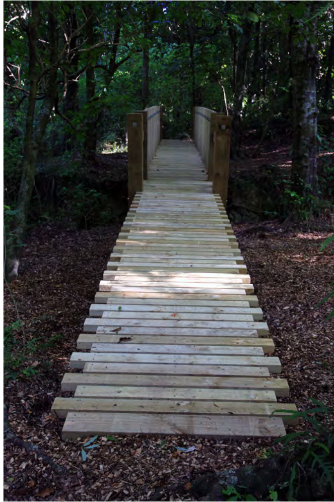
Walkway onto the Bridge
